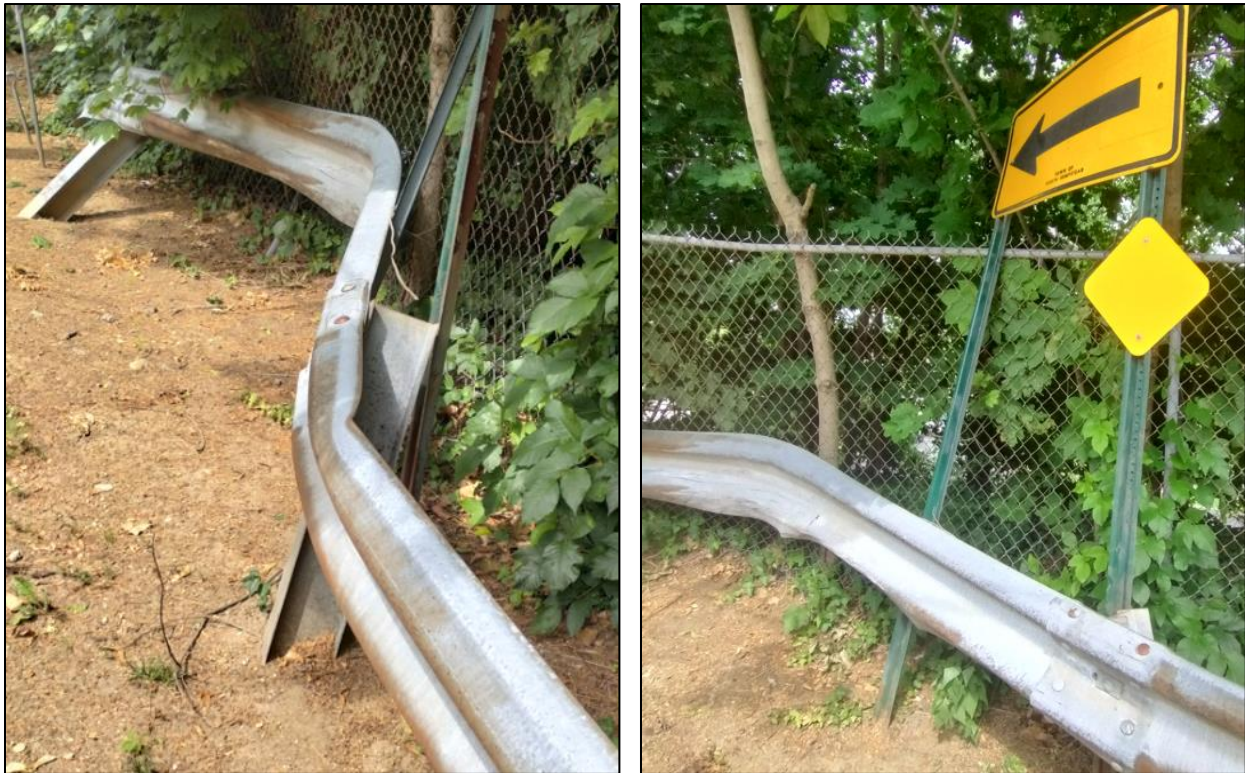
Photo 10: Misalignment of Existing Guiderail and Arrow Plaque
