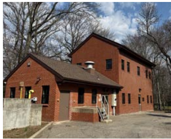
Eden treatment plant.
